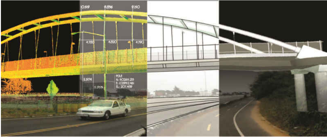
Figure 20: Image of bridge showing progression from scanned data on the left, automatic software distance calculations in the left-middle, 3D scan-to-model in the right-middle, and the normal picture of the bridge on the right (Leica Geosystems, 2010).
