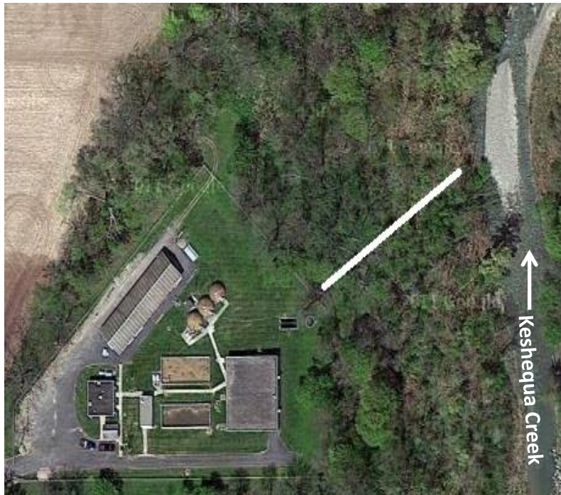
Figure 19. Nunda sewage treatment plant (WWTP) aerial view. White line shows ditch carrying effluent (approx. 56 m) into Keshequa Creek with arrow showing flow direction.
