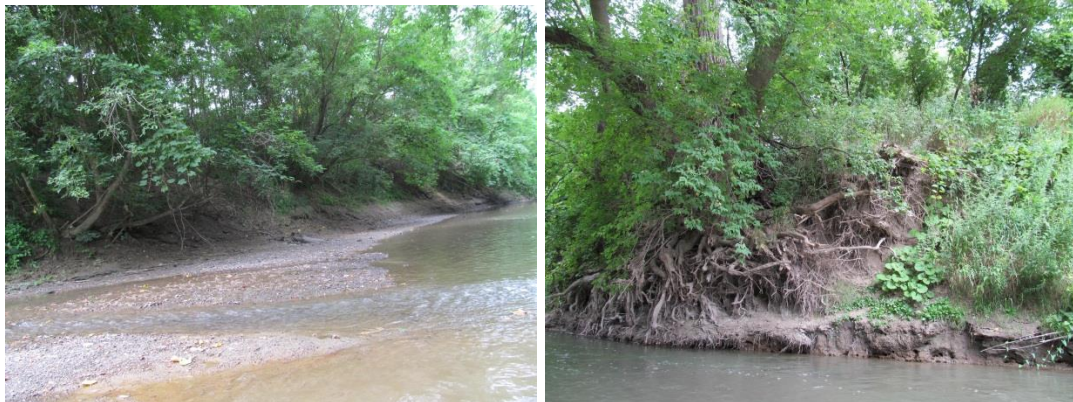
Figure E4. Groveland Flats site 8. The corn fields on either side of the stream in this reach limit the riparian zone to a thin (<20 m) strip. Trees were observed to be in the process of falling into the stream due to bank erosion.
