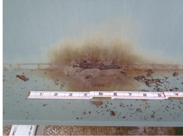
Figure 1.6: Weldment corrosion at the interstate bridge I 703: a) overview of the bridge, b) corrosion in a welded joint at the girder end, and c) corrosion in a fillet weld at the web-flange junction [10]
