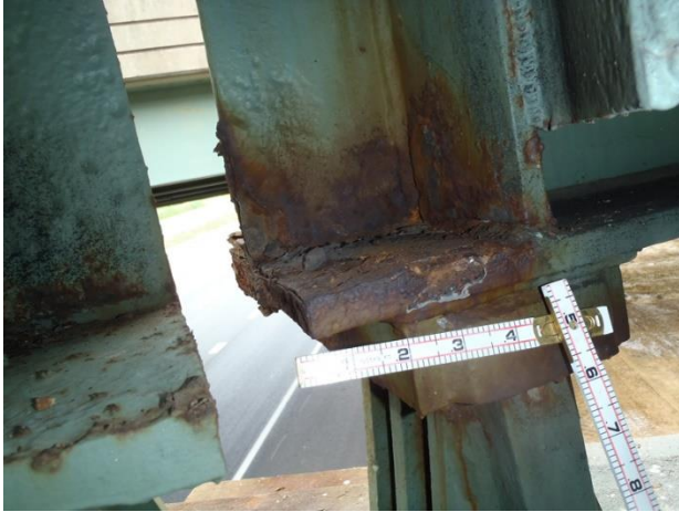
Figure 1.6: Weldment corrosion at the interstate bridge I 703: a) overview of the bridge, b) corrosion in a welded joint at the girder end, and c) corrosion in a fillet weld at the web-flange junction [10]
