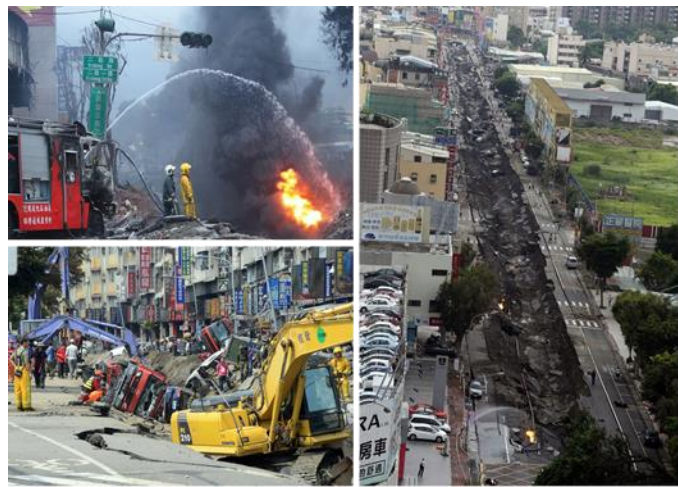
Figure 2.2: Corrosion-induced pipeline accident (Taiwan, 2014).
