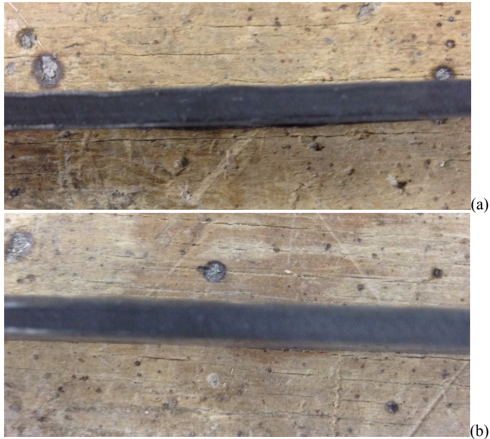
Figure 58. Close up of a damaged (a) and an undamaged (b) beam
