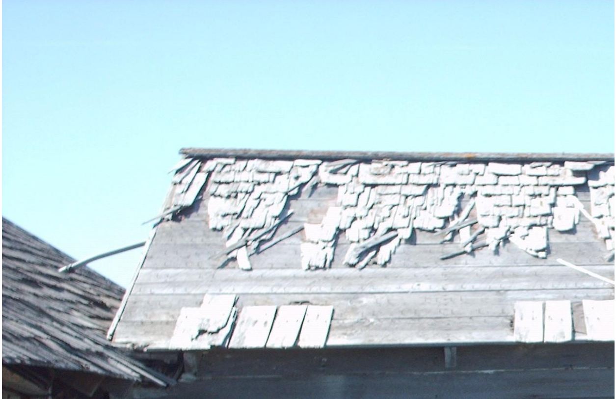
Fig. 6. Ruud home roof framing. Photo by author, 2009.
