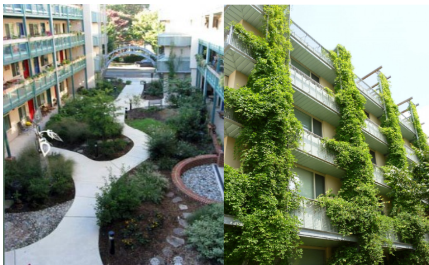
Eastern Village Cohousing: Courtyard (left), Front Elevation and Green Screen (Right)
