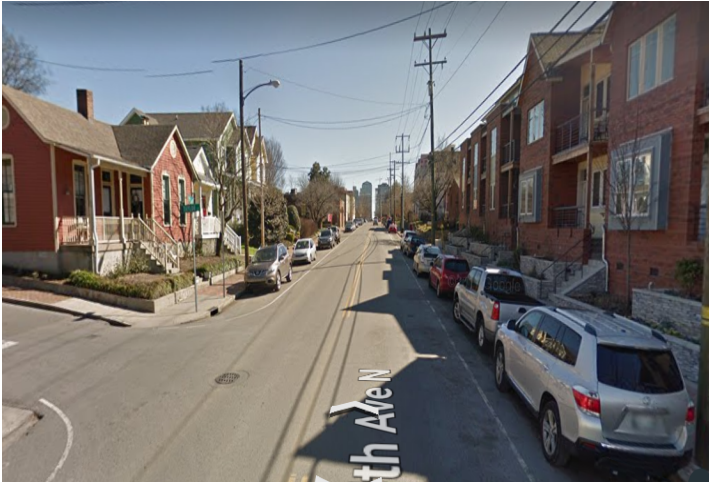
Street Facade on 5th Ave
