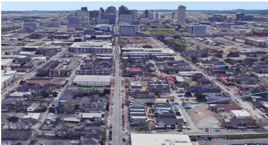
View of Subject Site Looking Towards Downtown Nashville
