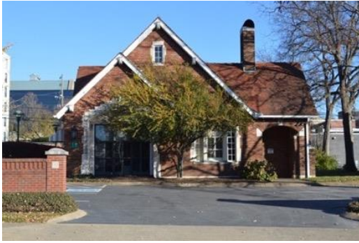
Former fire hall
