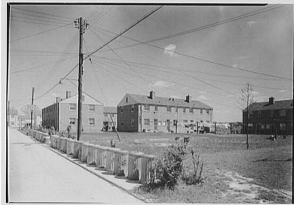
Rear view of one of the courtyards at Highland Dwellings. Gottscho-Schleisner, Inc., "Highland Dwellings, Washington, D.C. Refuse arrangements," April 28 th , 1944. Available at the Library of Congress website, https://www.loc.gov/item/2018743287/ (accessed November 29 th , 2019).
