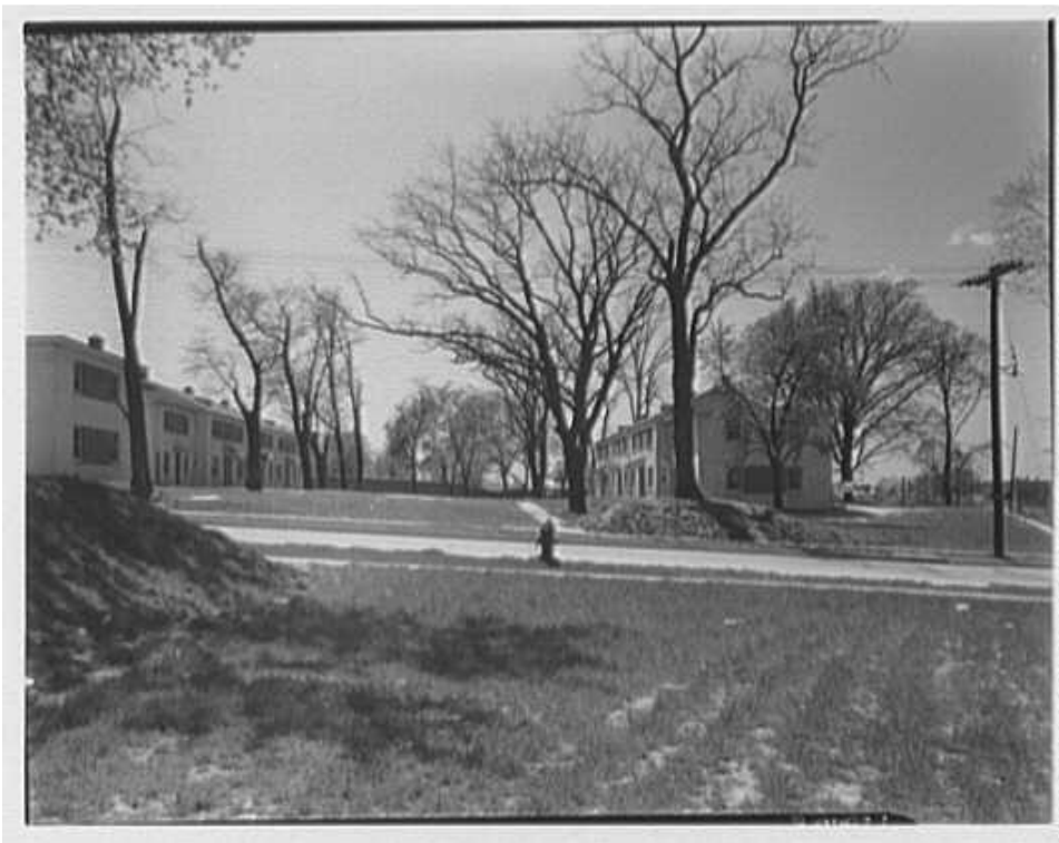
Another image revealing the sloped landscape of Barry Farms. The homes were kept fairly level on individual terraces, while the streets sloped noticeably downhill towards the Anacostia River. While the
