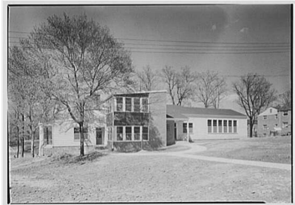
The Highland Dwellings Administration building. Note how the land clearly slopes from the right-hand side of the image to the left. Gottscho-Schleisner, Inc., "Highland Dwellings, Washington, D.C. Administration building," April 28 th , 1944. Available at the Library of Congress website, https://www.loc.gov/item/2018743292/ (accessed November 29 th , 2019).
