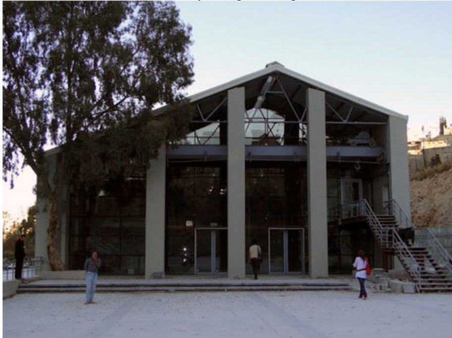
Figure 3-4, renovated Amman Electricity Hanger (Image © Rami Daher)
