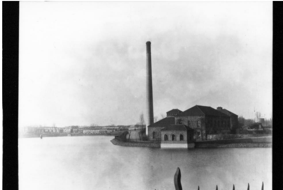
Figure 8: Filtration facilities, McMillan Reservoir, and smokestack, November 1916. Terrence Vincent Powderly Photographic Prints Collection. Catholic University Archives. http://hdl.handle.net/2041/61145
