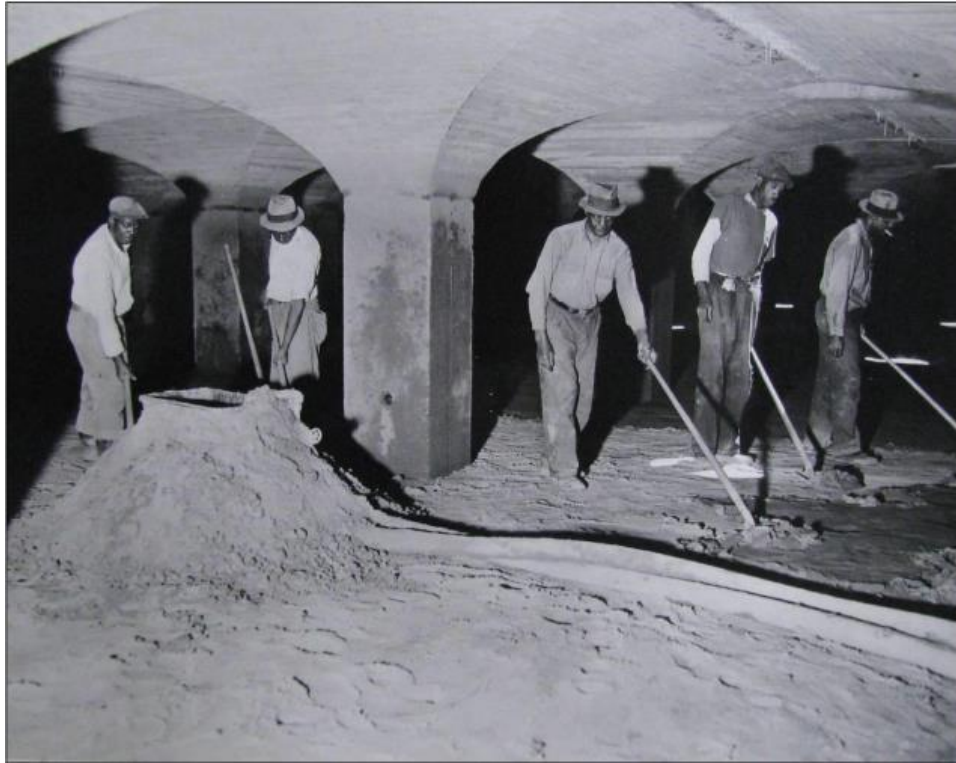
Figure 10: Workers removing sand for cleaning in filtration beds, 1938. Washington Evening Star , from June 12, 1938 article. Washington Historical Image Collection. Washingtoniana Division. Martin Luther King, Jr., Memorial Library.
