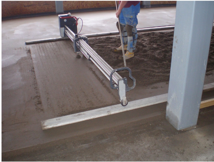
Figure 1. The self-propelled electrical screed levelling machine.
