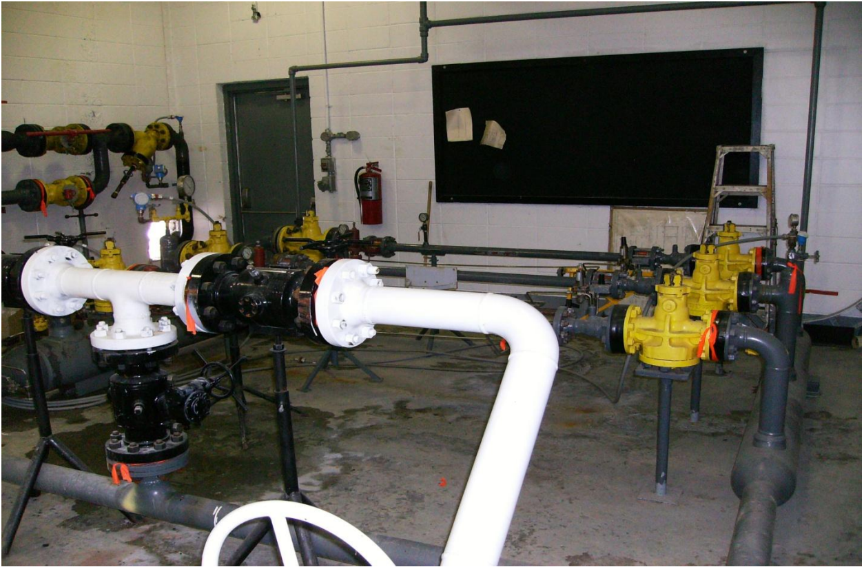
Figure 4.4 Glenburnie Pressure Regulation Valves
