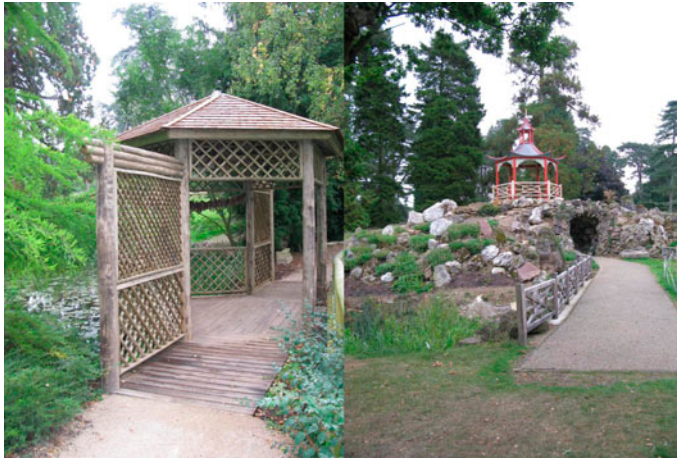
Figure 1. The Cone House (originally created 1805, restored and planted 2013) and Rockery Pavilion (originally created 1806, restored and planted 2004–2012) at Woburn Abbey Gardens, September 2013 © L. Veale.
