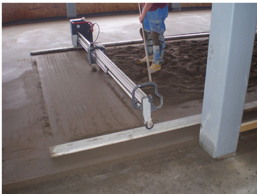
Figure 1. The self-propelled electrical screed levelling machine.
