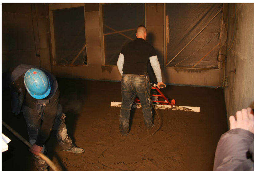
Figure 2. The manually moved electrical screed levelling machine.
