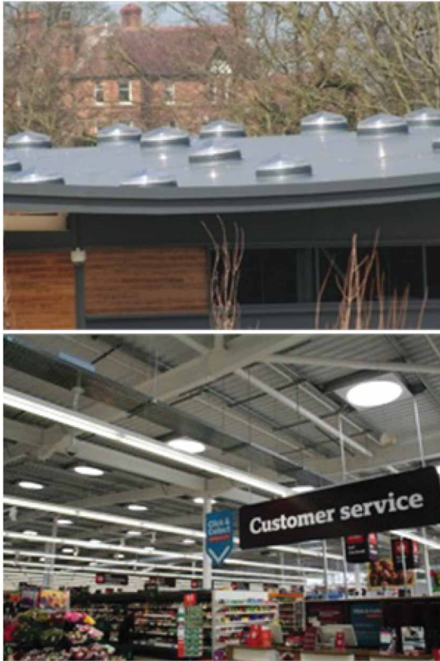
Figure 10. Roof lights of a supermarket opened in December 2012 (courtesy of Monodraught Ltd).
