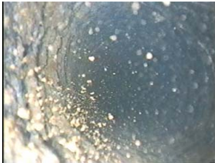
Figure 3-5: Biofilm present all over the wellbore at 29.3 meters below top of casing in WWFS.
