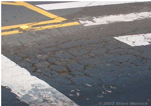
Figure 1. A typical area of fatigue distress [10]. Figure 2. Typical rutting distress [10].
