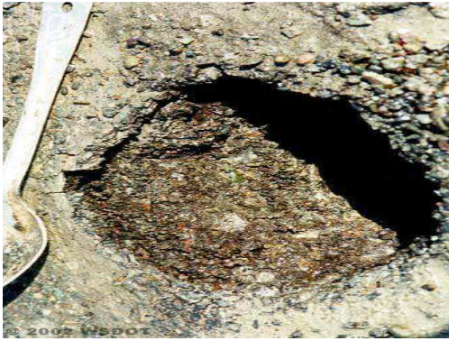
Figure 3. A small stripping distress [10]. Figure 4. A typical thermal effect on road [10].
