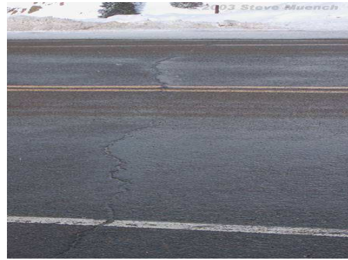
Figure 3. A small stripping distress [10]. Figure 4. A typical thermal effect on road [10].
