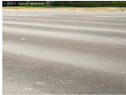
Figure 1. A typical area of fatigue distress [10]. Figure 2. Typical rutting distress [10].
