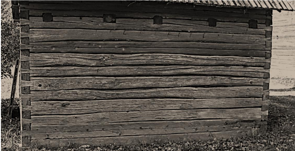
Figure 5.2 Dovetailed Broad Axe Hewn Construction. (Photo by Author)
