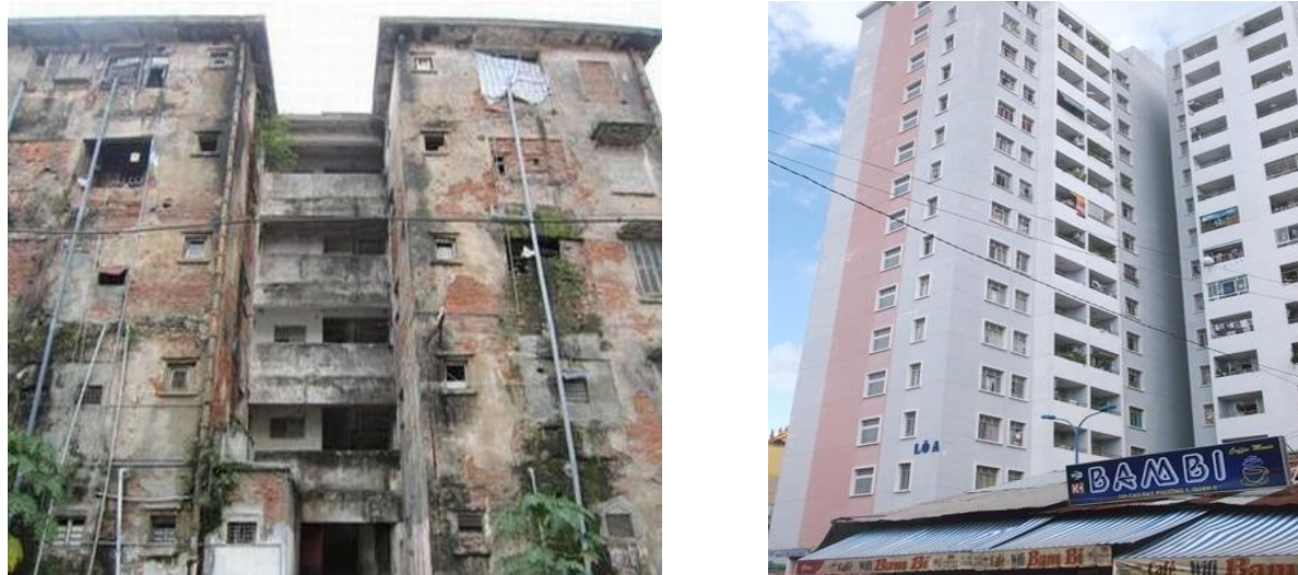
Figure 2.2 Apartment blocks project N 0727
