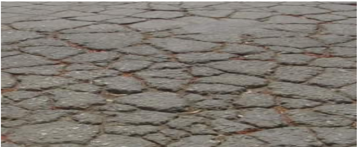
Figure 9. Alligator Cracking [48].
