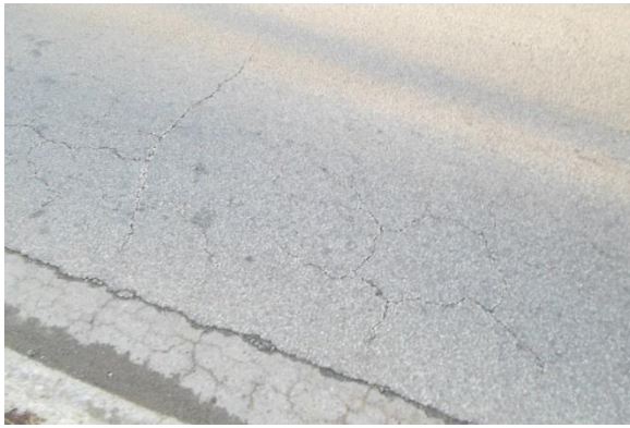
Figure 79. Evidence of Fatigue Temperature cracking in the field.
