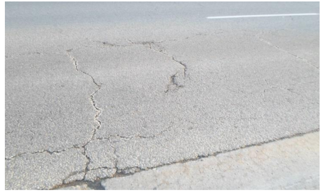
Figure 79. Evidence of Fatigue Temperature cracking in the field.
