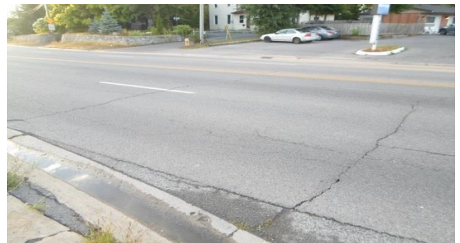
Figure 78. Evidence of Low Temperature cracking in the field.
