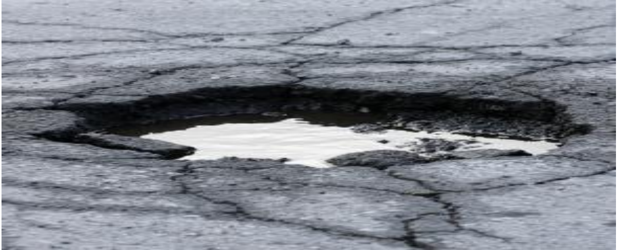
Figure 10. Potholes [49].
