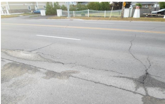
Figure 78. Evidence of Low Temperature cracking in the field.
