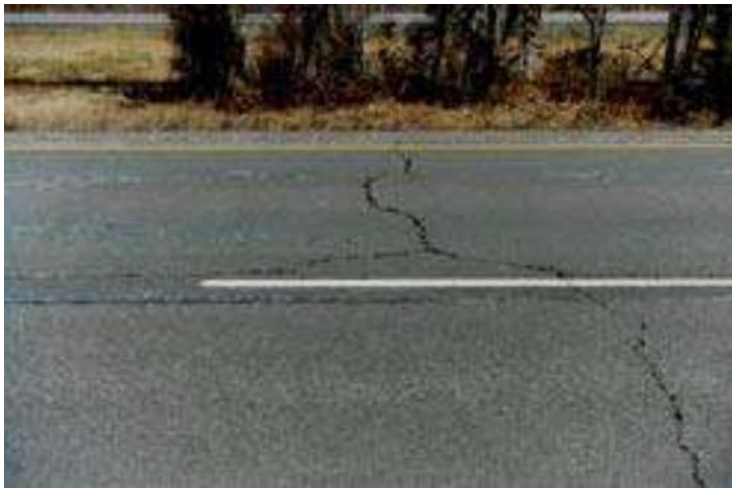
Figure 1.4 Low temperature cracking [21].
