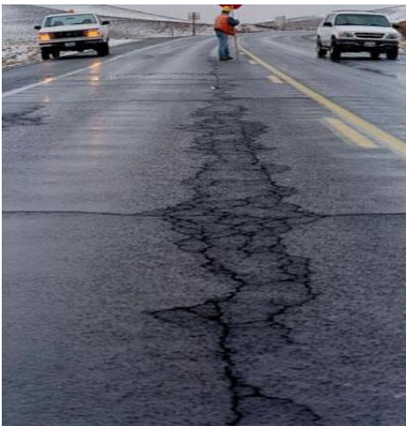
Figure 1.6 Stripping in pavement [21].
