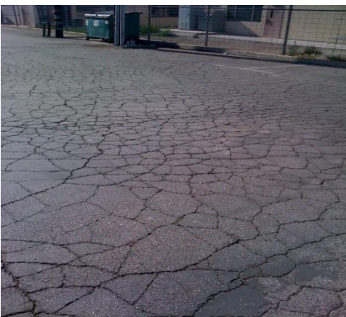
Figure 1.3 Fatigue cracking [21].
