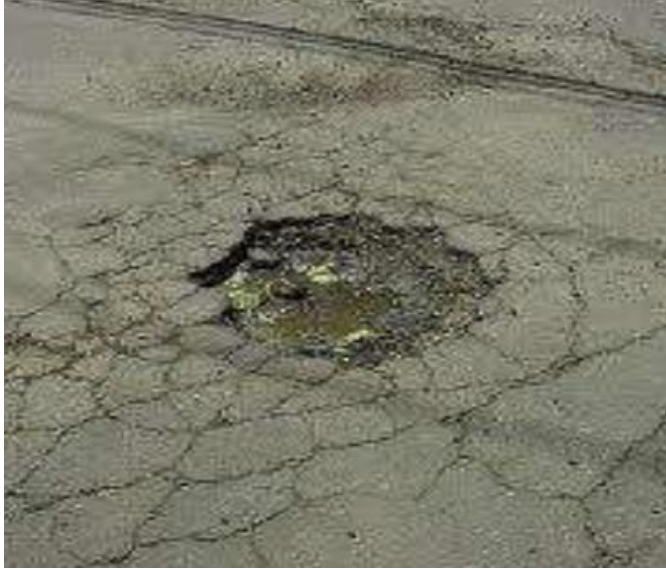
Figure 1.5: Moisture damage [11].
