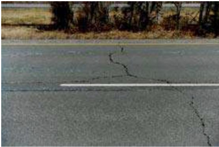
Figure 1.4: Thermal cracking [10].
