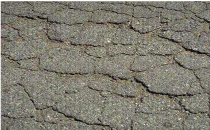
Figure 1.3: Fatigue cracking [8].
