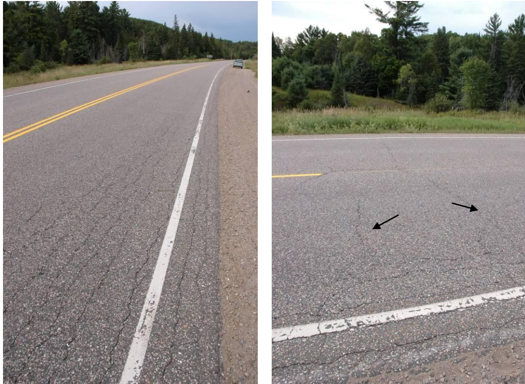
Figure 17. Typical surface condition of Highway 41 contract near Denbigh.
