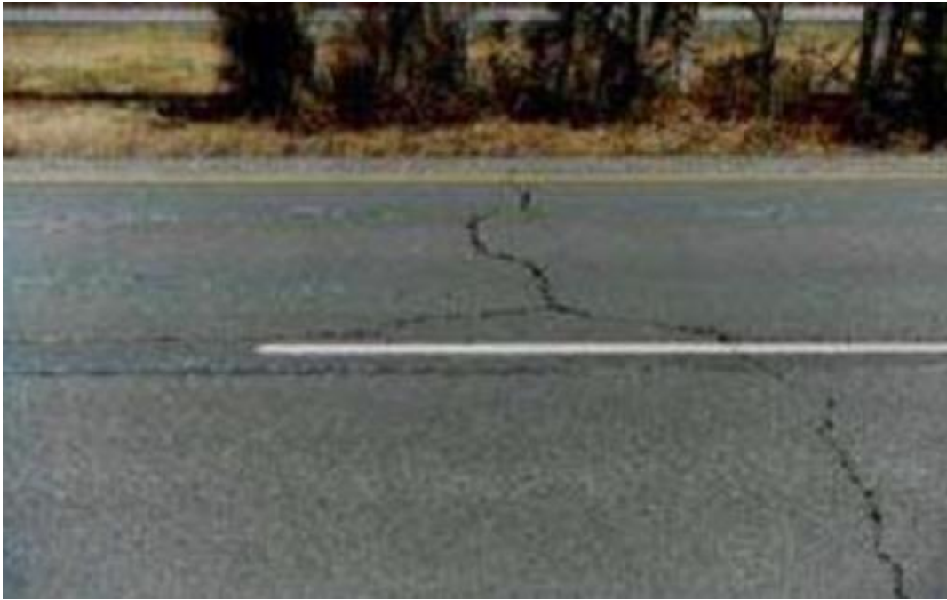
Figure 2.4: Thermal cracking [38].
