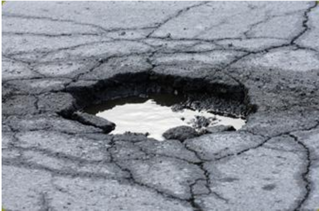
Figure 2.5: Moisture Damage [42].
