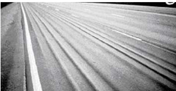
Figure 1c. Ruts on the wheel path
