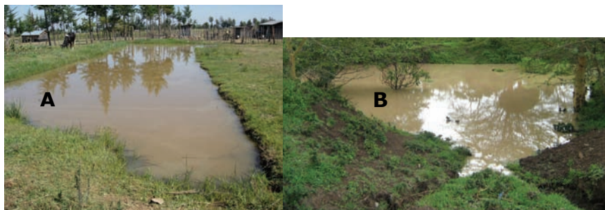
Figure 7.11: RWH storage (macro-systems) for SIR (A) and livestock watering (B) in the downstream part of the basin.
