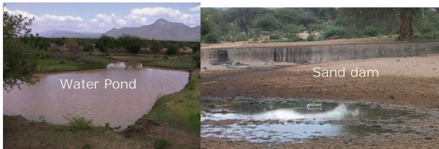
Figure 7.13: RWH storage systems for watering livestock found downstream of the basin
