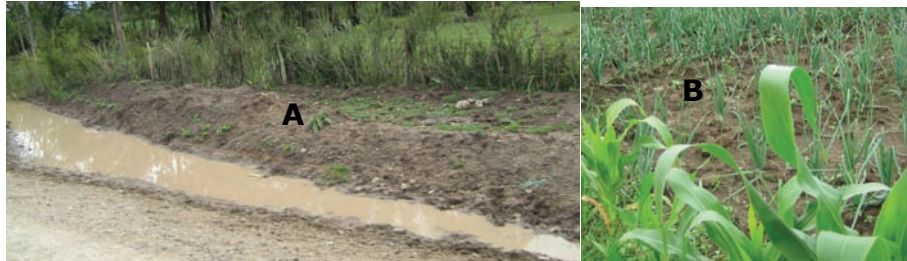
Figure 7.8: Directing runoff from a road reserve (A) to a RWH storage (Macro-systems) for SIR downstream (B).
