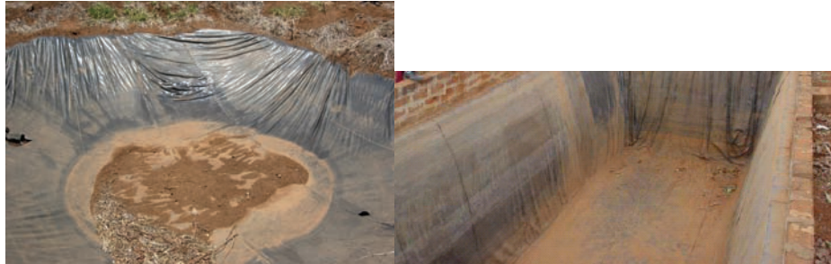
Figure 7.12: Measures for minimizing water losses from RWH storage systems for SIR in the lower part of the basin.
