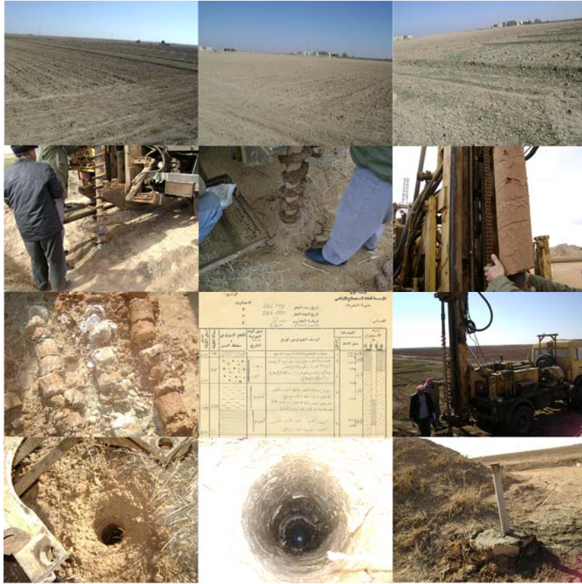
Figure 3.3: Scenes from the study area. Drilling a piezometer. The soil core of a borehole. A sample of a boreholes conducted by the General Organization for Land Reclamation, Ar-Raqqa, Syria.
