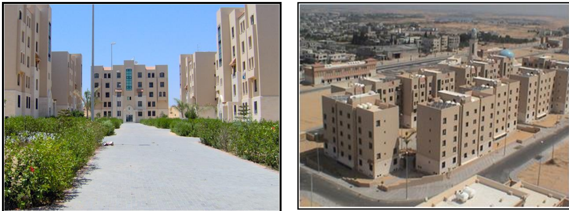
Figure (2. 14): Views of urban courtyard at Sheikh Zayed housing project Source: MPWH, (2014)
