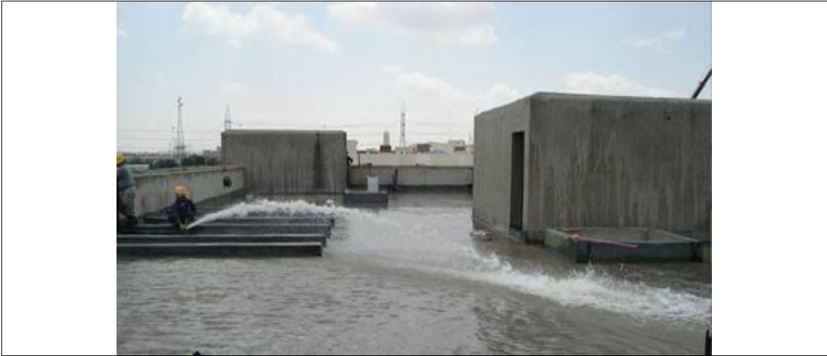
Figure 4.20: The process of inspecting waterproof with submersion method
