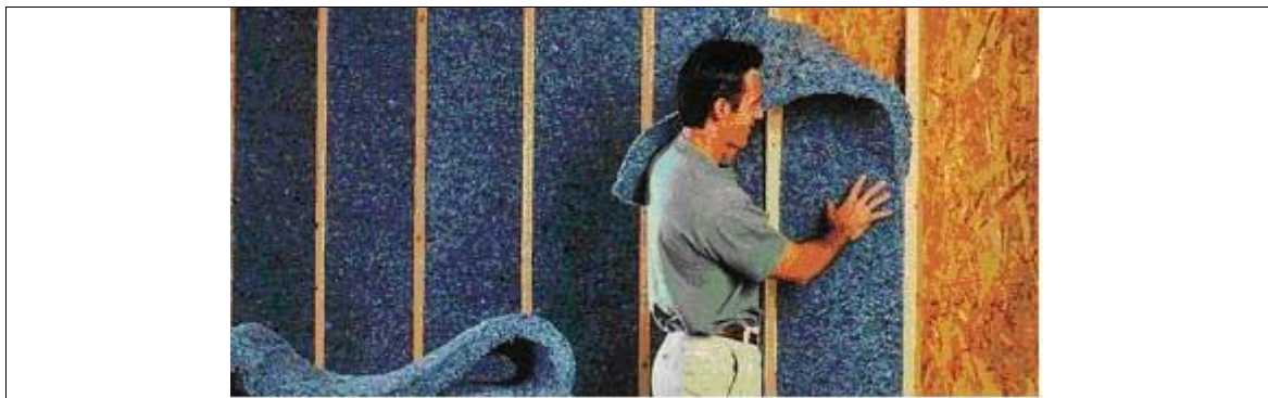
Figure 4.8: Natural cotton insulation
