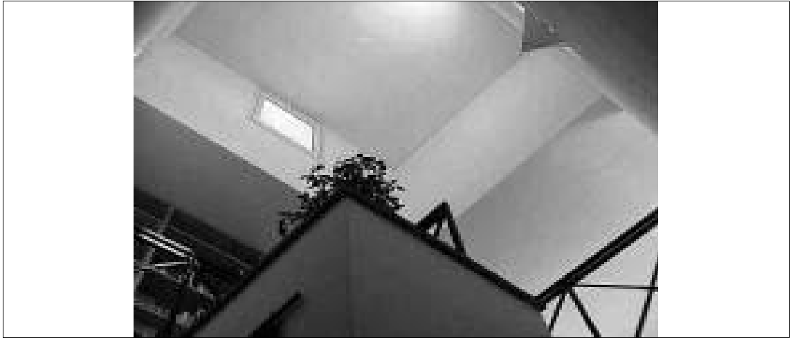
Figure 5.10: Windows on upper levels enable ventilation (cross, stack, and suction) during summer season nights Source: (Roaf, 2007)
