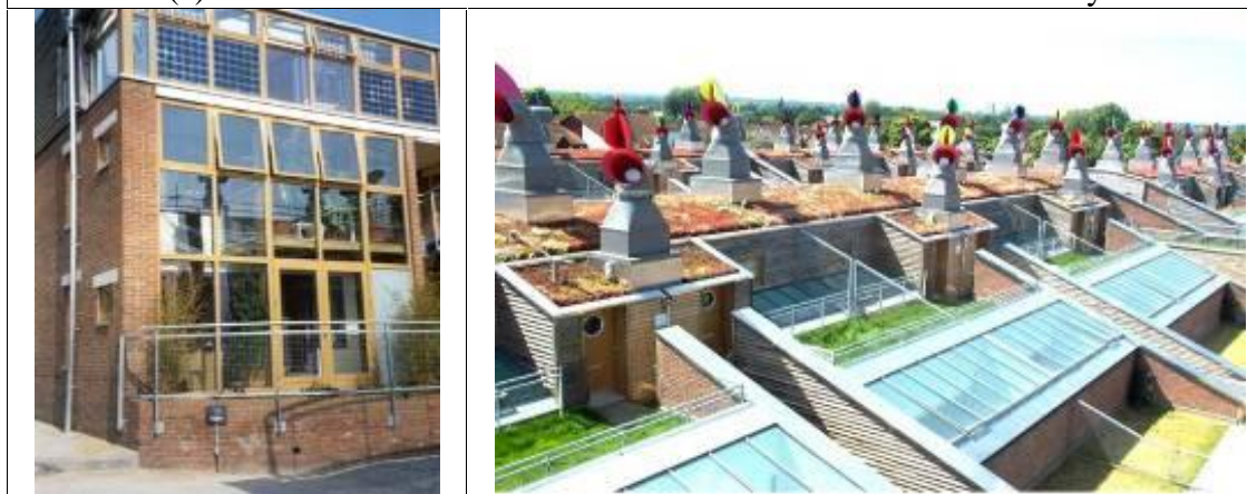
(b): Multifunction Glass Areas (Solar Gain, Natural Lighting, and Ventilation).
