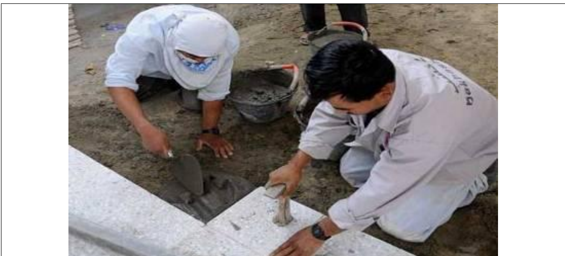
Figure 4.21: The process of installing tiles over the protective concrete layer
