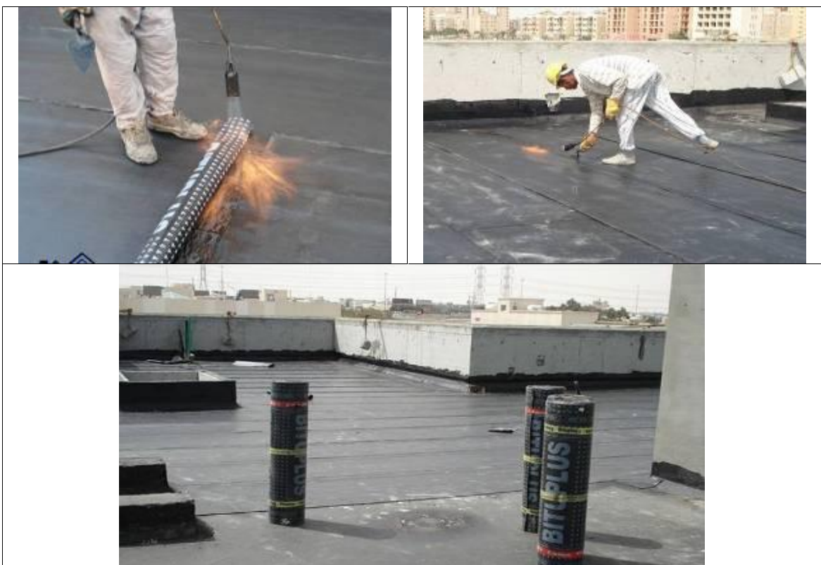
Figure 4.19: The process of fixing waterproof rolls over the foam concrete
