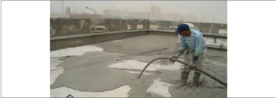
Figure 4.18: The process of pouring a layer of foamed concrete on the roof
