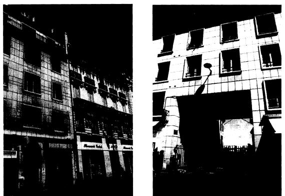
Figure 2.07 & Figure 2.08 - Orléans: proportional systems from undamaged buildings are carried into the reconstruction project (left) while architectural elements recalling a French classical past are incorporated in the new city (right).
