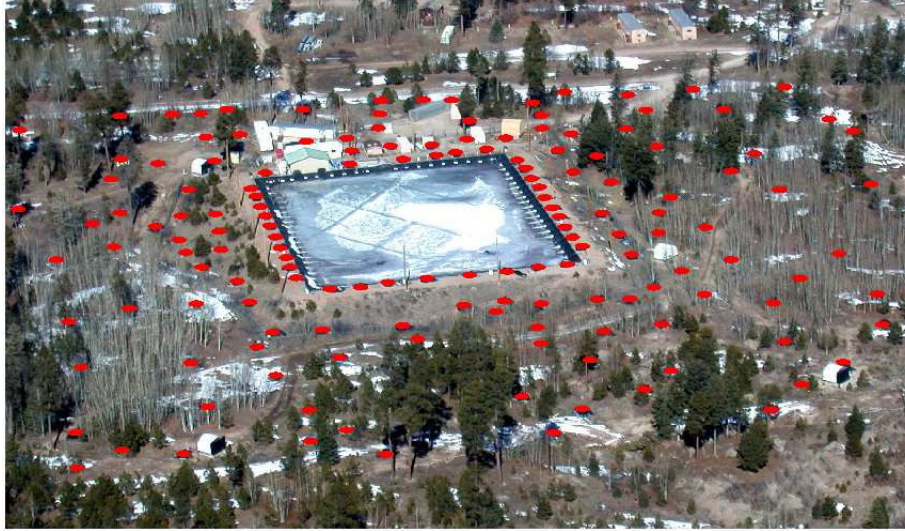
Figure 2.3: Overhead view of pond with red markers where tanks were placed in 2004. Image taken from [3].
