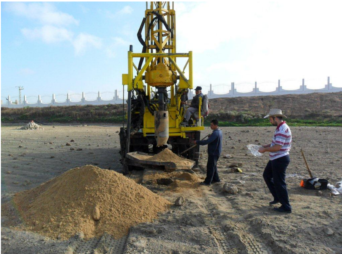
Figure (4-2): Drilling method using Rotary Auger
