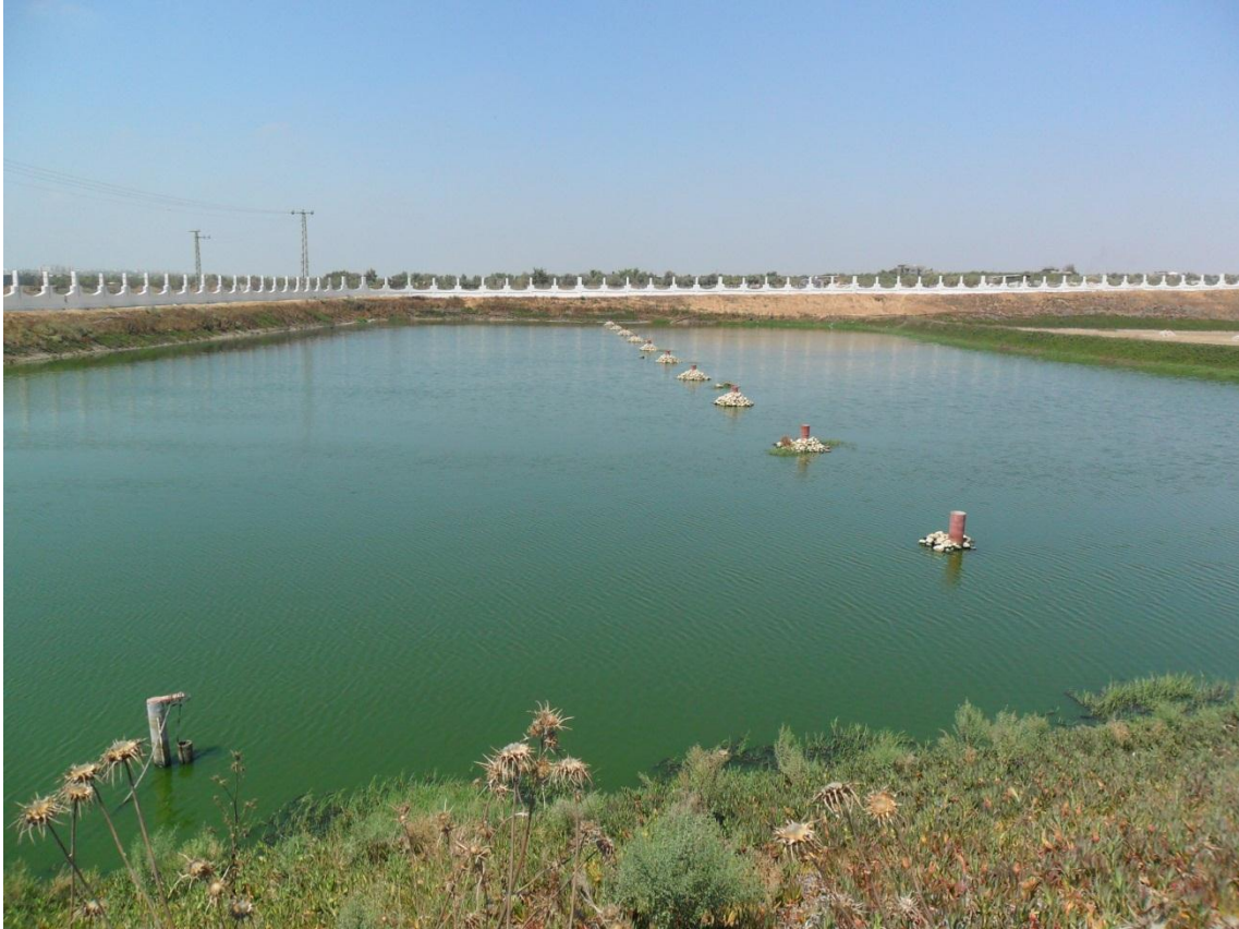
Figure (3-8): General view for infiltration basin IB1(July, 2013)
