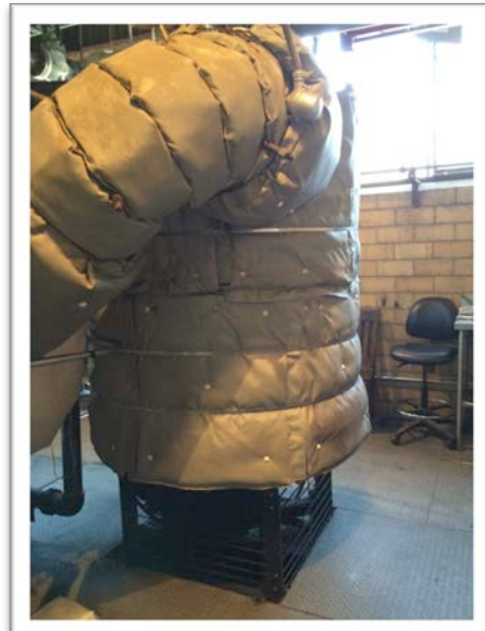
Figure 2.4 : Outer view of the gasifier
