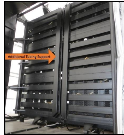
Figure 9.4: Support tube added to edge of outer doors
