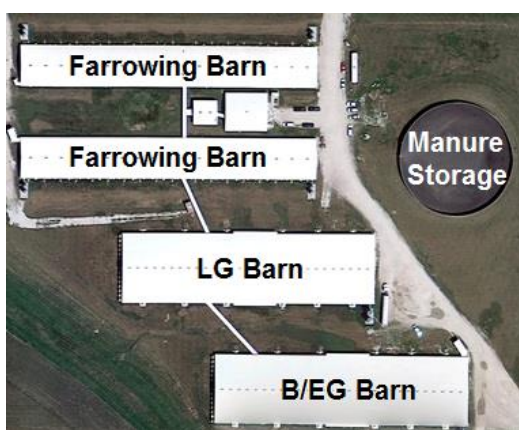
Figure 2.1. The breeding-gestation-farrowing facility aerial view for the farm monitored in a study evaluating gaseous emissions from a swine operation.
