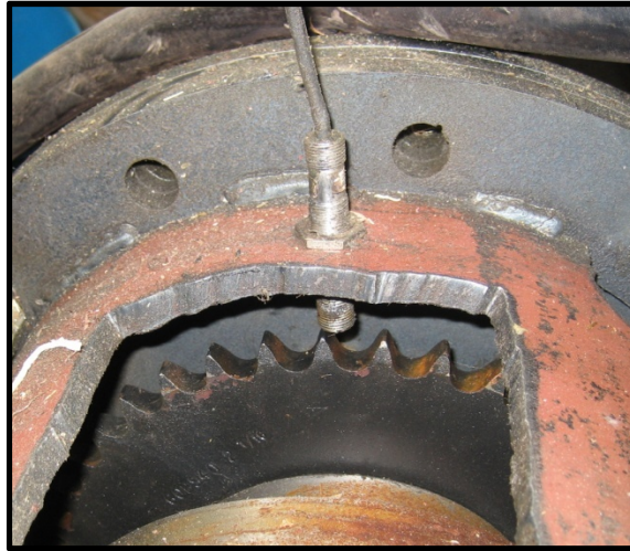
Figure 8. Shaft mounted sprocket and magnetic auger speed pickup sensor for the compaction system.
