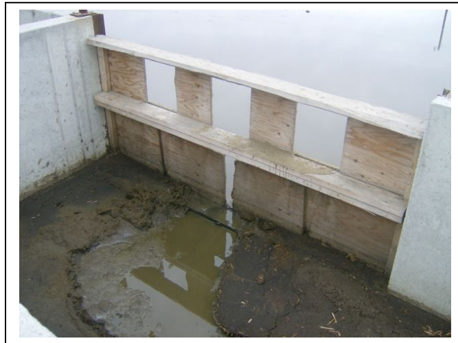
Figure 10: V-notch SSB outlet at Northwest IA 2
