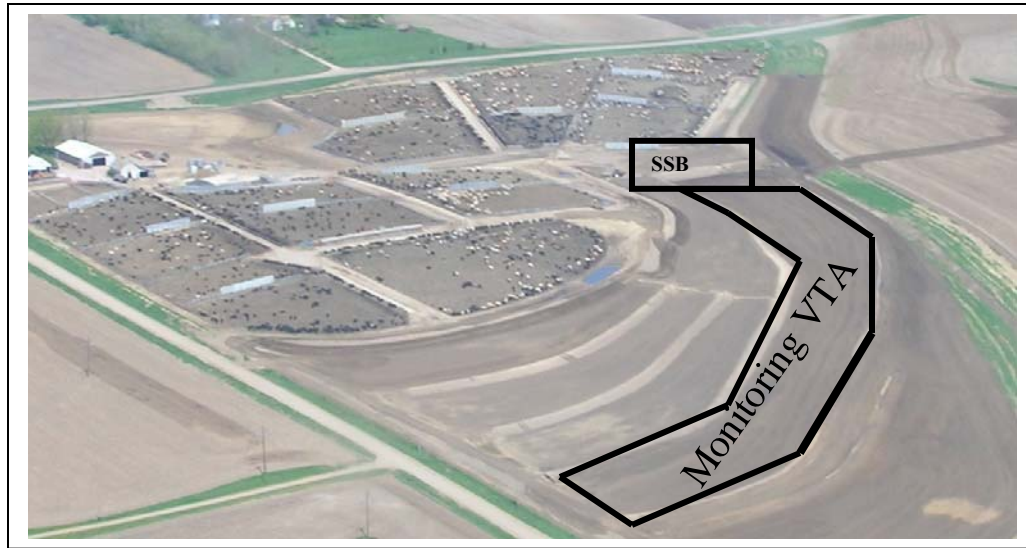
Figure 8: Aerial view of the Northwest IA 1 VTS with highlighted research VTS portion
