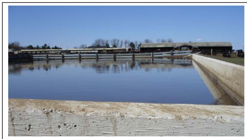
Figure 44: Water backed up in the feedlot while the SSB still has room available at the sides
