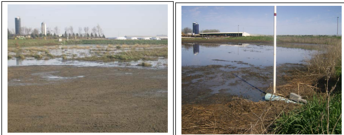
Figure 34: (L to R) Solids accumulation in one half of the VIB towards the inlet and standing water in the other half towards the outlet in 2007 at NW IA 2
