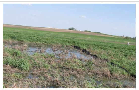
Figure 6: Geotextile flow spreader in the Central IA 1 VTA
