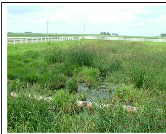
Figure 28: Ponding present at to top half of the Central IA 2 VTA
