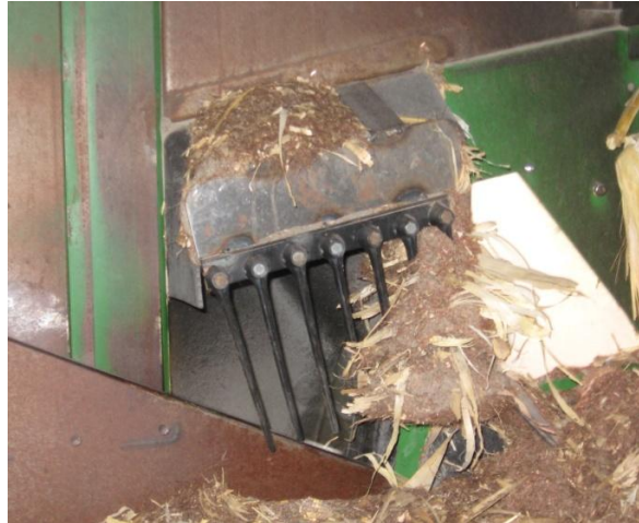
Figure 9. Guards were installed over the air vents to prevent cobs from exiting the machine before the chopper.
