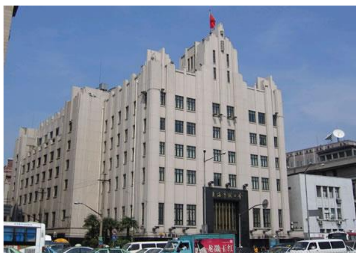
Fig.6.5 Communication Bank Building (CB building)
