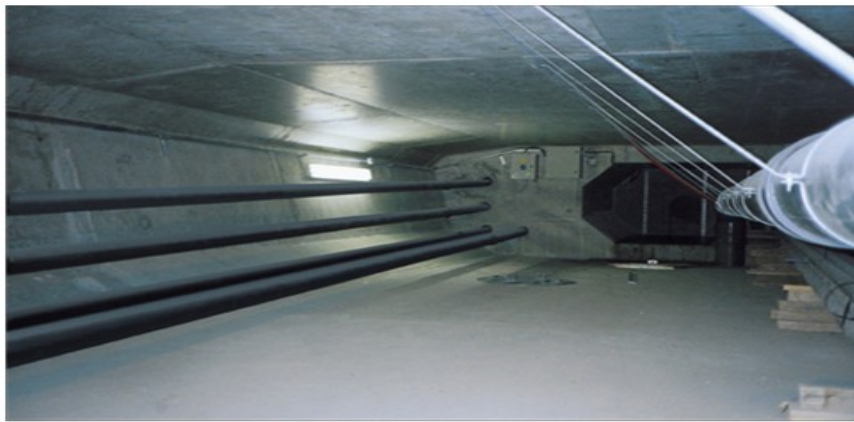
Figure 1.1: External Post-Tensioning in a bridge ( www.cclint.com )
