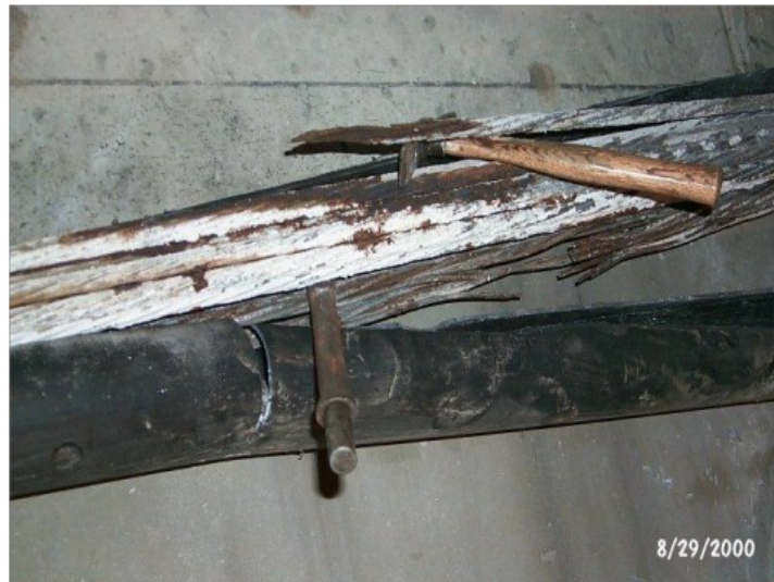
Figure 1.4: Cracked duct showing severely corroded strand ( www.dot.state.oh.us )
