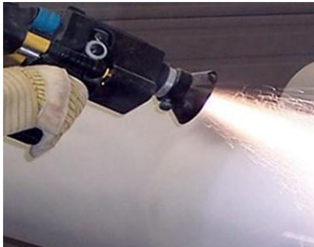
Figure 7.1 Metallizing of steel pole.
