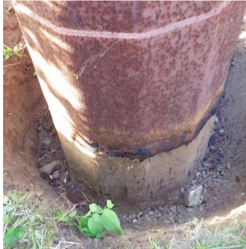
Figure 7.2 Sacrificial WS sleeve installed at base of WS pole.
