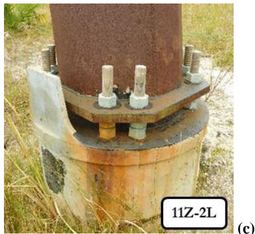
Figure 3.29 Visual assessment of poles at Site 5: (a) discolored patina, corroding fasteners, and vegetation build-up around Pole 8Z-2R; (b) uniform patina but corroding fasteners on Pole 11Z-6R; and (c) uniform patina and GS fasteners on Pole 11Z-2L.
