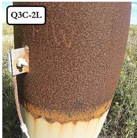
Figure 3.8 Corrosion prevention measures seen on Site 2 poles, including GEC link to grounding rod and magnesium anode connection.
