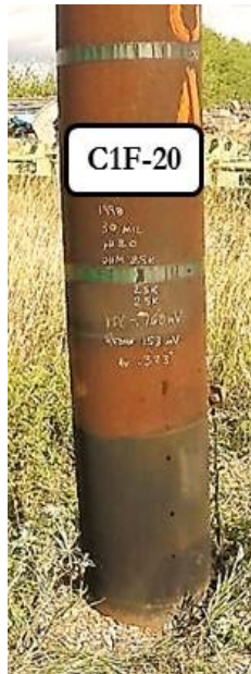
Figure 3.3 Ground-level view of Pole C1F-20 at Site 1.
