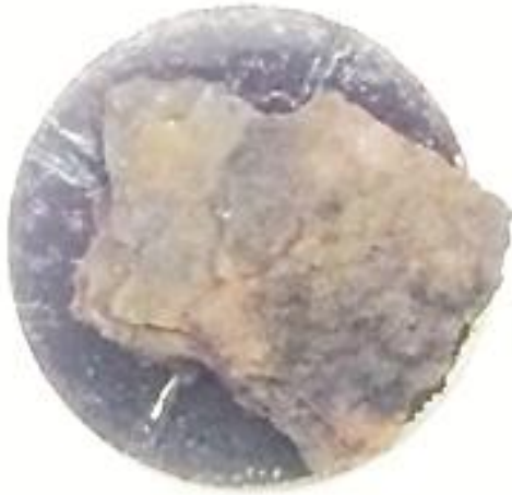
Figure A.13 Loose rust sample from GS fastener region of Pole 8Z-2R at Site 5.
