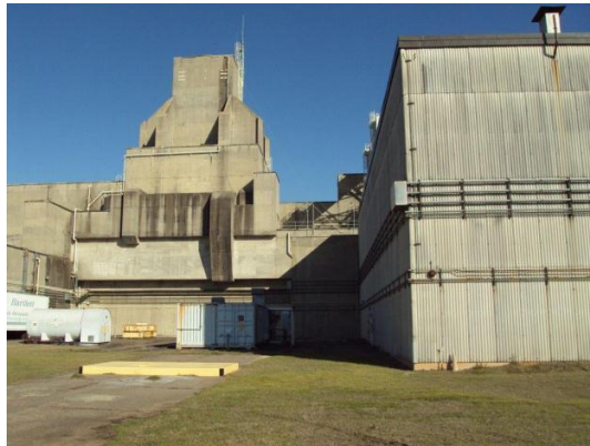
Figure 5.1 Reactor building 105-C at the Savannah River Site.
