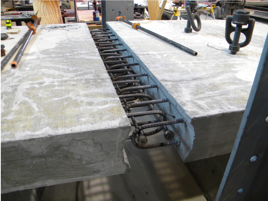
Figure 3.13: View of completed joint prior to pour
