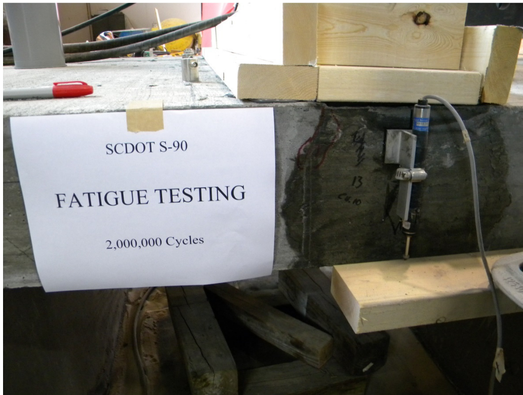
Figure 3.22: Joint condition following fatigue testing
