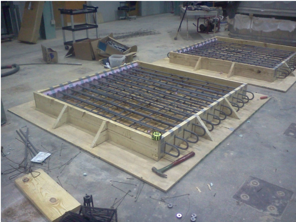
Figure 3.7: View of tied rebar with lift inserts
