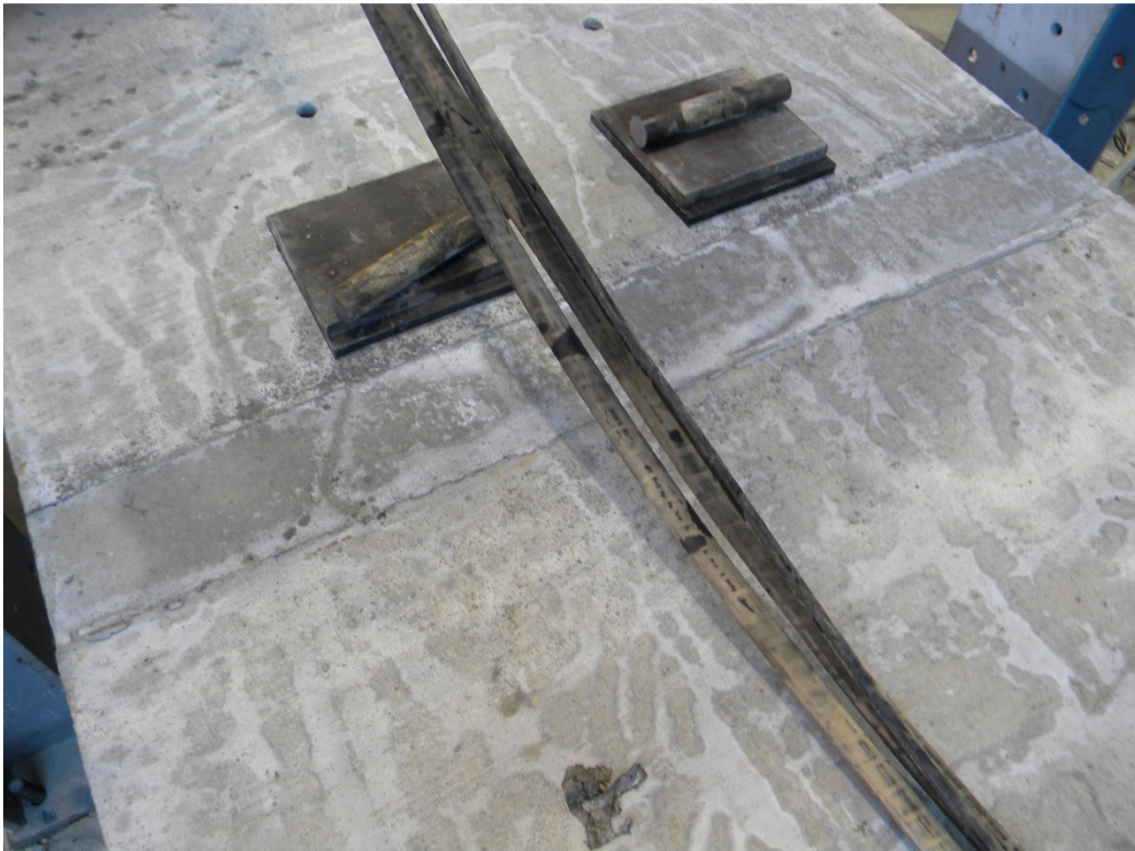
Figure 3.14: Joint following closure pour
