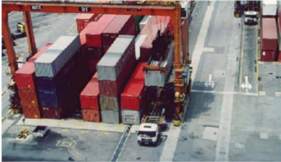
Figure 2.5 Rubber tyred Gantry crane. (Murty et al, 2005)
