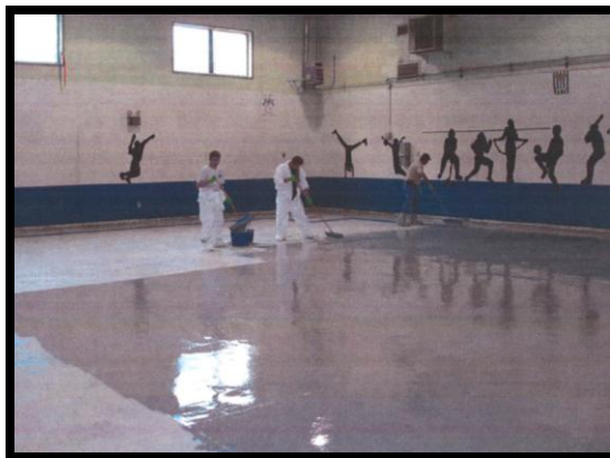
Figure 4. 1: Decontamination efforts in the gymnasium (EPA photo, 2008).
