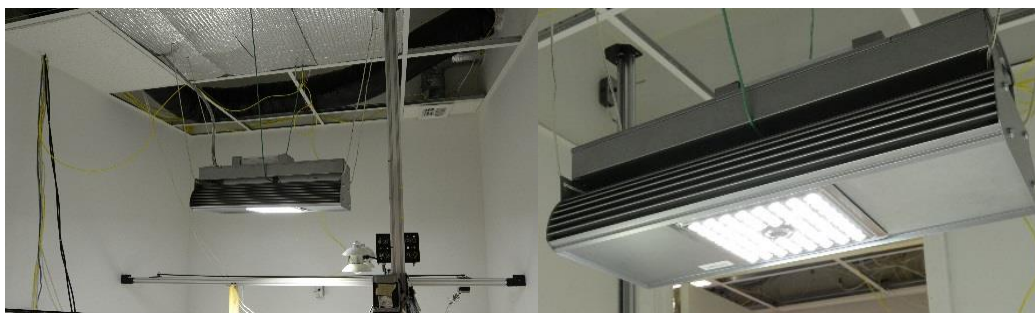
Figure 7-5 Rectangular-Shape High-Bay with Direct Optics
