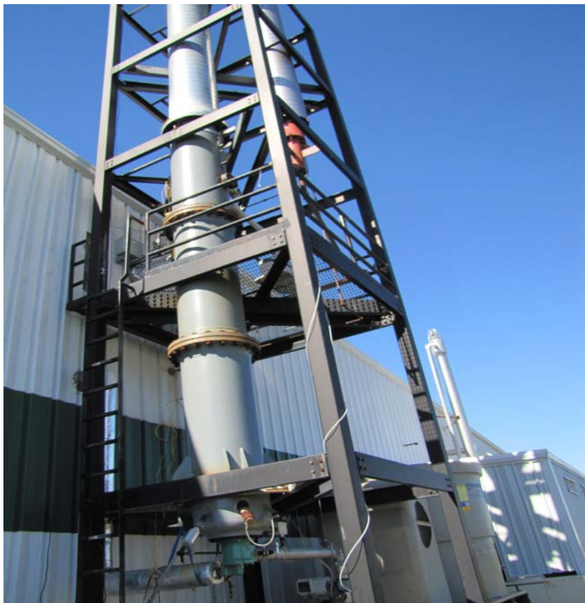
Figure 3.2 Combustion chamber
