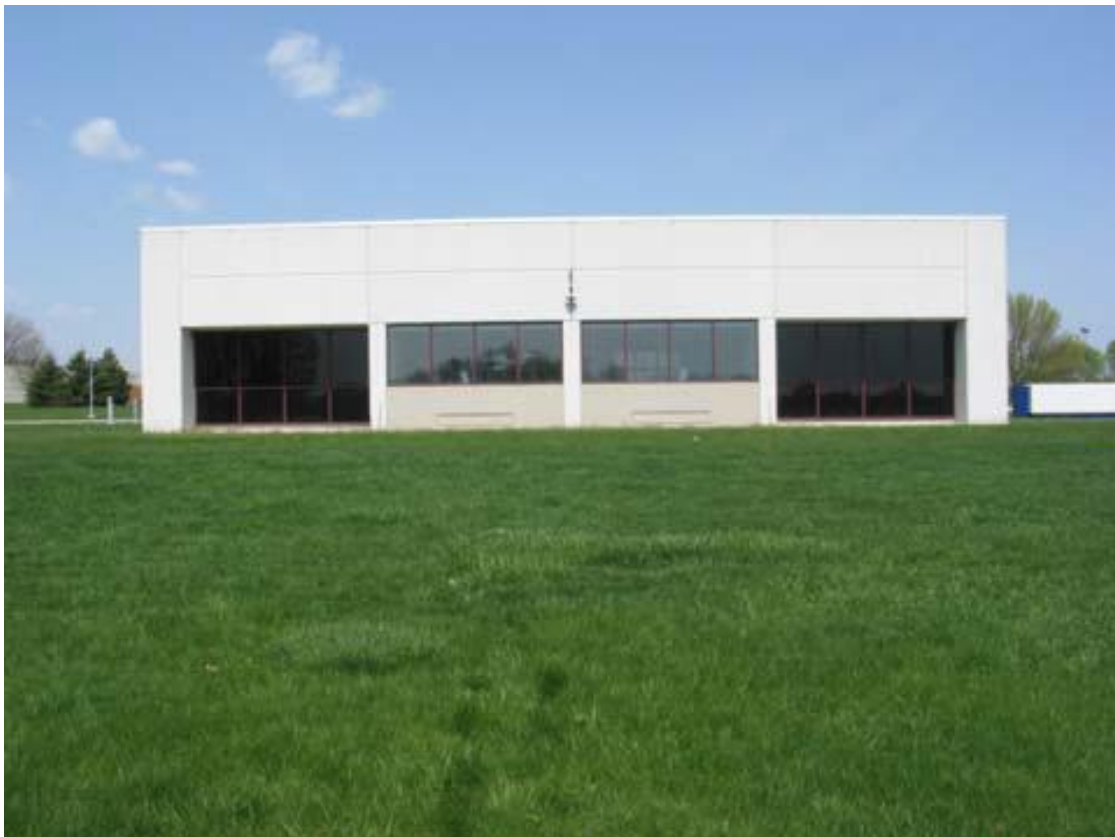
Figure 24: South A and B test room exterior walls
