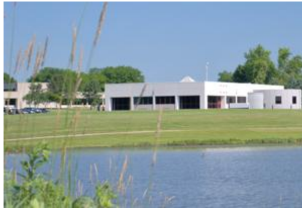
Figure 1: Iowa Energy Center Energy Resource Station (ERS)
