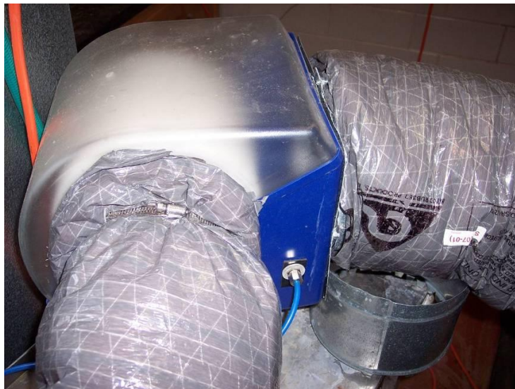
Figure 104. Humidifier typical for residential furnace
