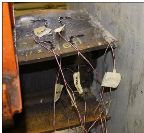
Figure 5.19 Retrofitted abutment buckling of base section
